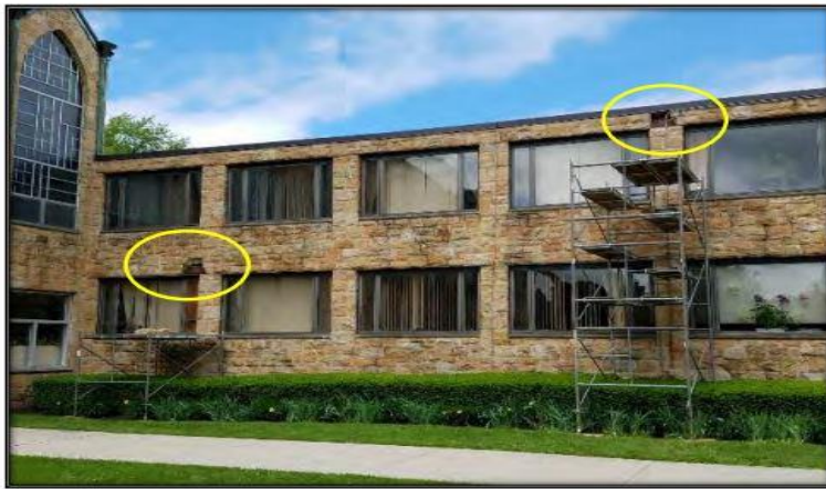
Photo 1 – Locations of Stone Removal to Observe Steel Lintels
